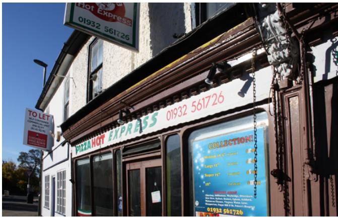
Remnants of a historic shopfront (retractable canopy, consoles, pilasters)
