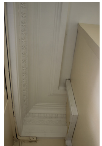
Examples showing a suspended ceiling and modern subdivision
